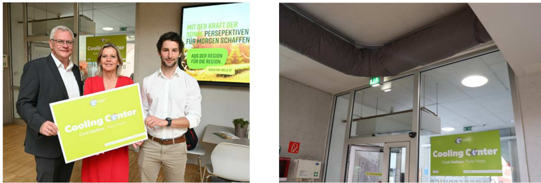
Figure 2: Left: Opening Ceremony of the Cooling Center, right: Distribution of the cool air via textile ducts (© Sandra Koeune)
