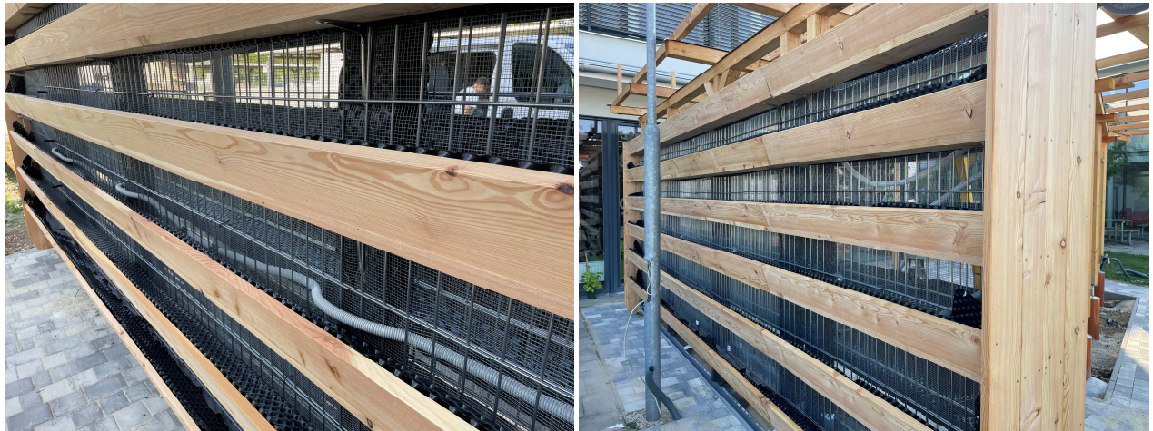
Fig. 9 and 10: Ground construction/substructure of the EVAPO+ transpiring green wall within the outdoor classroom at the Middle School in Strasshof
