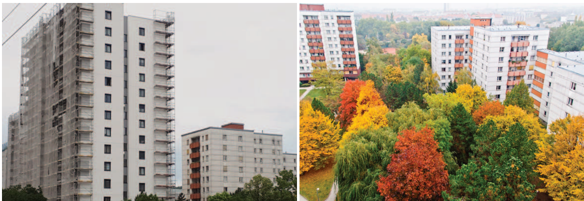
Figure 2: The final stage of building refurbishment at Hauffgasse
