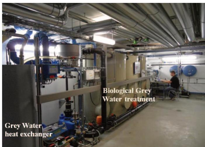
Fig. 7: Heat exchange and biological treatment of separated Grey Water in an apartment house in Berlin (Germany). Foto: H. Lehn
